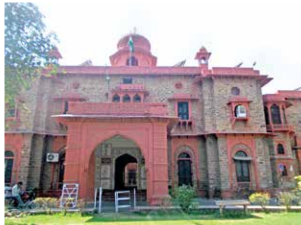
Ajmer Municipal Corporation Heritage Building
